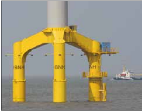
▲ Offshore wind turbine leveling: Enerpac's synchronous lifting system was the solution for leveling support cross pieces on 80 wind turbines.
