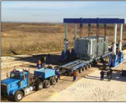
Transformer Installation with a Hydraulic Gantry
